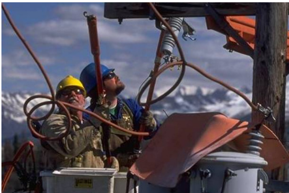
Image courtesy of Anchorage Municipal Light & Power.
